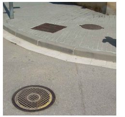
Tapes circulars registre pous pluvials i residuals.
